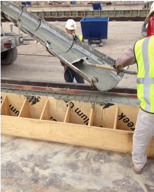
(a) Placing Concrete
