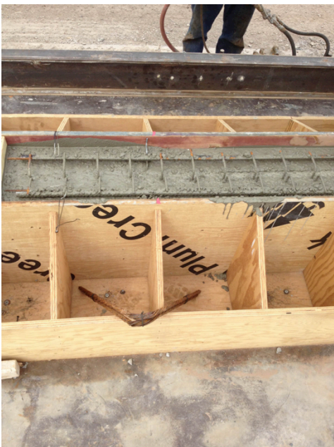
(b) Vibrating Concrete
