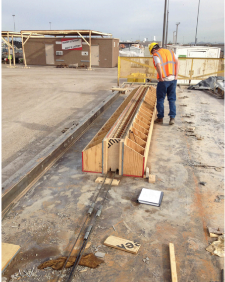
(a) Checking Formwork
